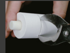
Final removal with a plaster nipper
